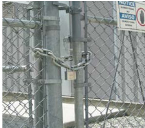
Perimeter gates and fences
